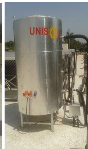
Fig. 2. Hot water storage tank
