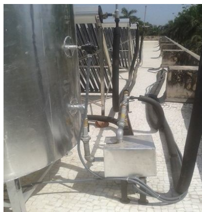
Fig. 3. Pipeline for hot water circulation from tank to the incubation room
